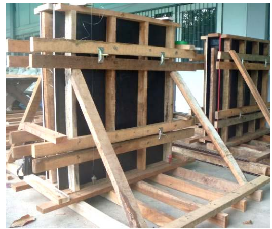
Figure 2 Wall formwork
